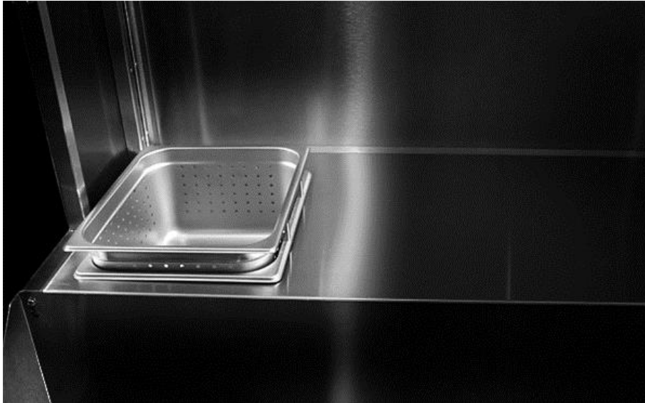
Picture 4. Gently drop the sink or ice bin in the top shelf hole. Ice bin shown here.
